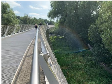
The Living Bridge
